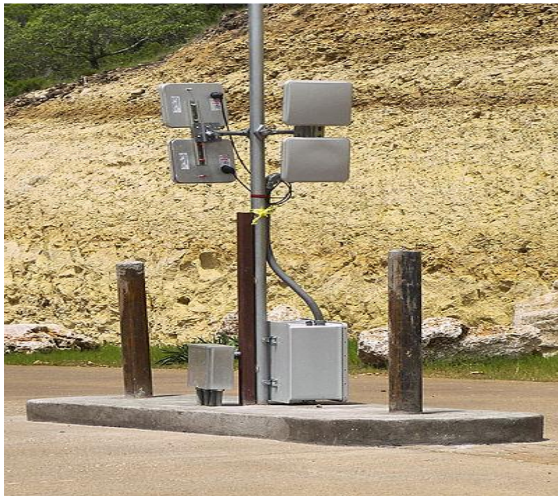
Picture 2: RFID antenna for container access that are transported by truck Source: http://en.wikipedia.org/wiki/Radio-frequency_identification
